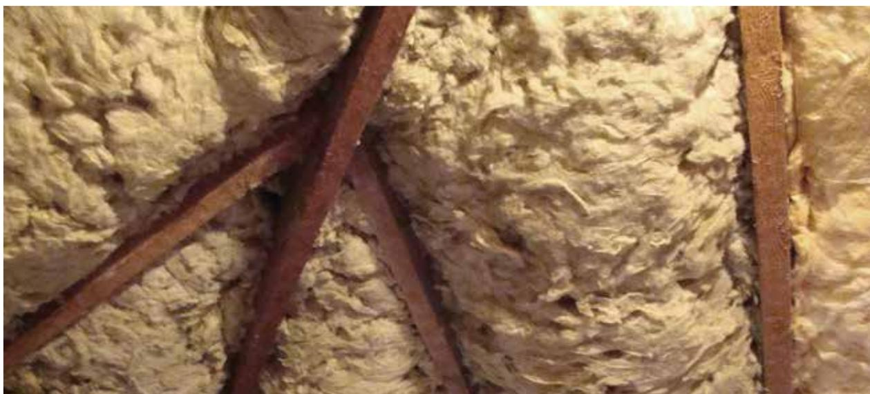
Wool based roof insulation.
